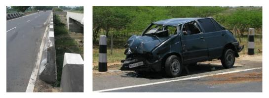
Figure 15. An Open Ended Bridge Wall Built Very Close to the Roadway (left) was the Cause of a Truck Crash; and a Crashed Car which Impacted the Concrete Poles (right).
