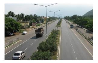
Figure 4. Typical Section of NH45 with Wide Median and Paved Shoulders.
