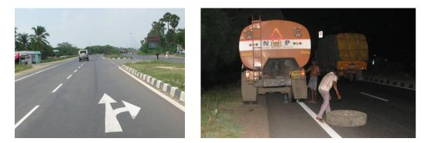
Figure 13. Vehicles Proceeding Straight or Taking a Turn Share the Same Lane at a Gap in Median (left); and a Truck Parked Partly on the Road for Repairs (right).
